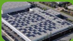
Photovoltaic systems at North America QA-Lab
